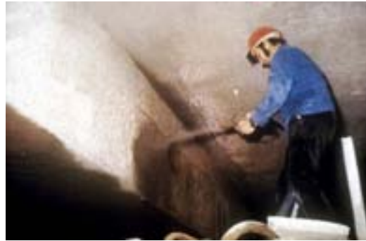
Figure CS1.3 Repairing elements with guniting (sprayed concrete) (Courtesy DBV, Germany)
