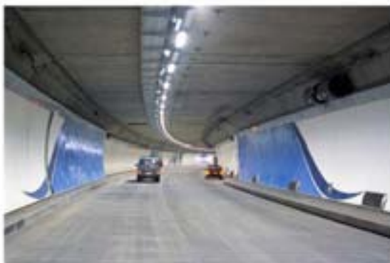
Figure 1.4: Concrete tunnels and road surfaces will stand up to the extreme fire conditions encountered in tunnels.
