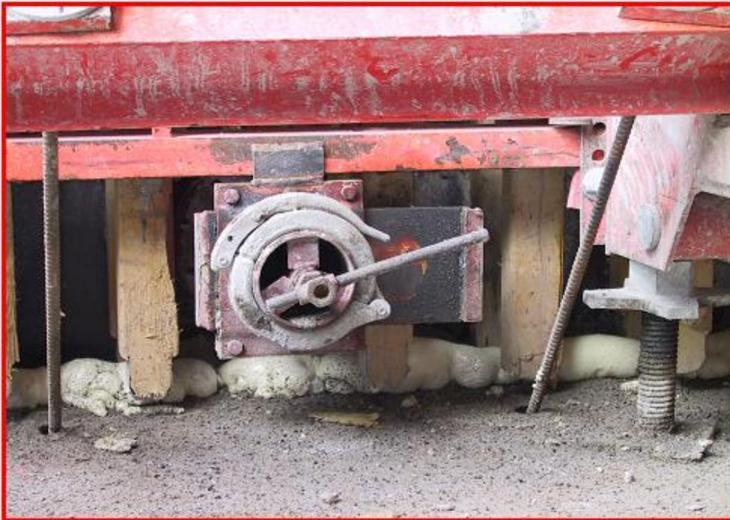
**Figure 10.1:** After pumping from the bottom, protruding concrete can be pushed flush with the inner surface of the formwork via a special spindle or the surface made good after removal of the formwork.
