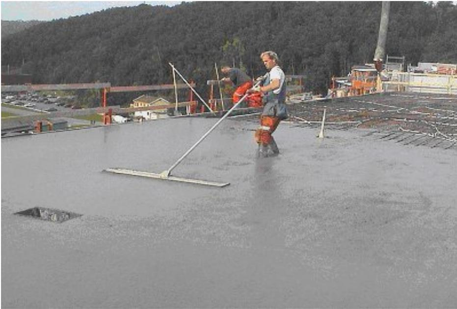
**Figure 11.1 Levelling SCC with a skip float**
