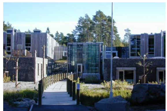
Figure 5f: Kvernhuset Youth School in Fredrikstad, Norway. An energy efficient building utilising ready mixed concrete to obtain energy savings and featuring many other sustainable solutions. (Courtesy of Photographer: Terje Heen - Municipality of Fredrikstad)
